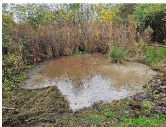
Pond Restoration at Manor Farm Community Centre
